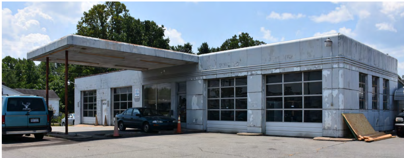
Service Station, northeast oblique
